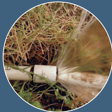
Temporary above-ground installation that has become permanent. It leaks around 3,500 m 3 /year.
